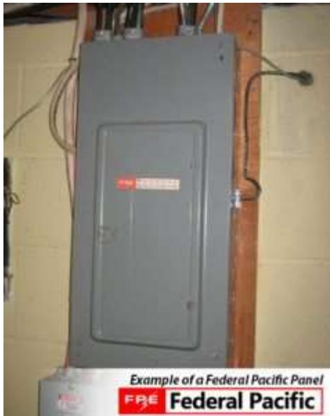
A Federal Pacific Electric (FPE) circuit breaker panel can appear to be working properly for years. BUT experts warn that if a Federal Pacific Electric panel experiences an overcurrent or short circuit, it may not keep the electrical circuits from overheating and could possibly pose a fire hazard.
